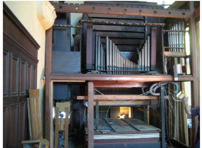
The bellows before removal.
